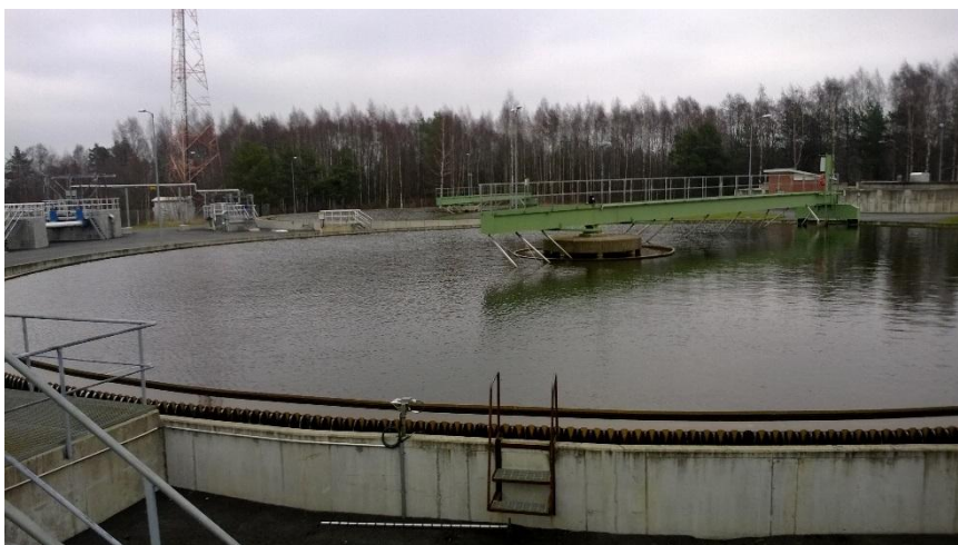
Picture 3. In the final sedimentation phase the water looks like clear (Eliisa Punttila)
